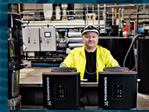
Scott Curran, Maintenance Team Leader, William Grant & Sons' Girvan Distillery
